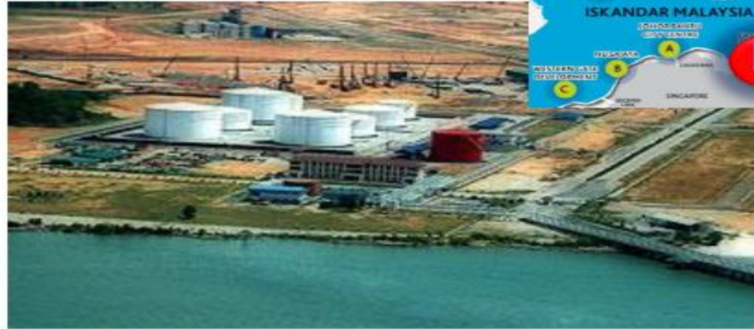
TANJUNG LANGSAT INDUSTRIAL COMPLEX
