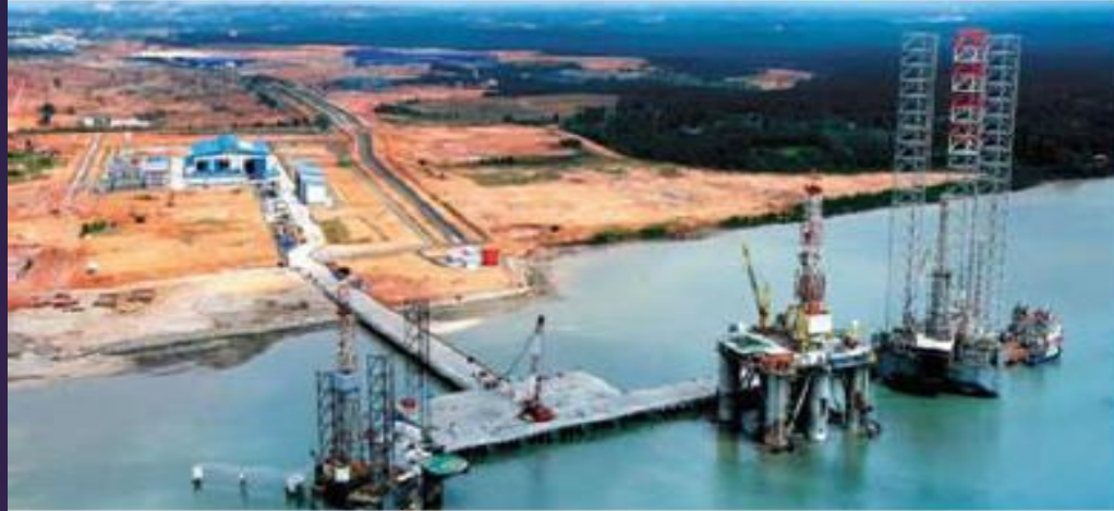
TANJUNG LANGSAT TERMINAL
