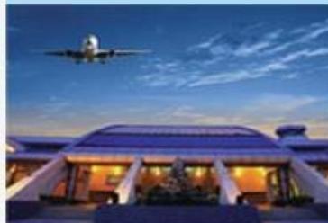
Senai International Airport
